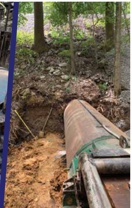
MULDRAUGH, KENTUCKY 120' Emergency Culvert Replacement 48" casing
