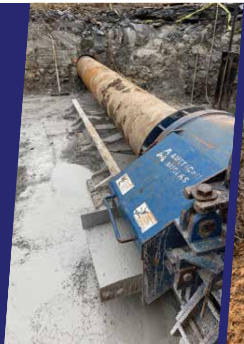
CHARLESTOWN, INDIANA 80' Gravity Sewer Bore 24" casing Solid Limestone
